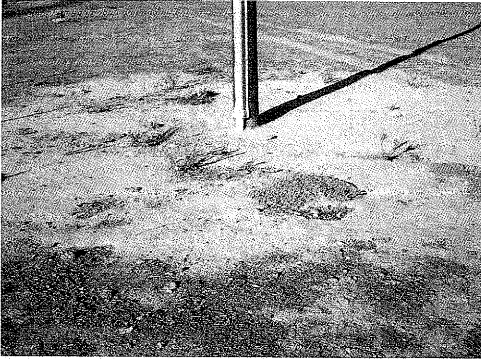
Paso 160 Project – Basin 2
